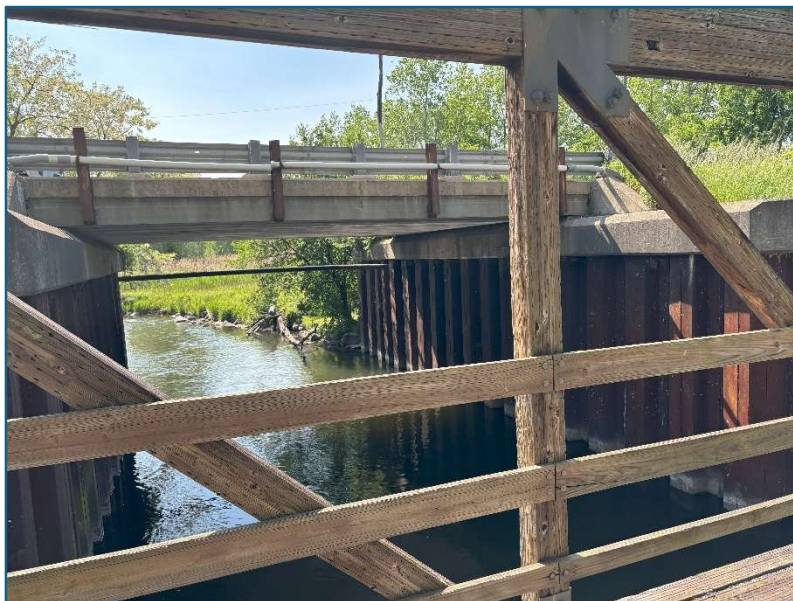
Figure 6.9: Clinton River under Adams Road, north of River Trail Drive
