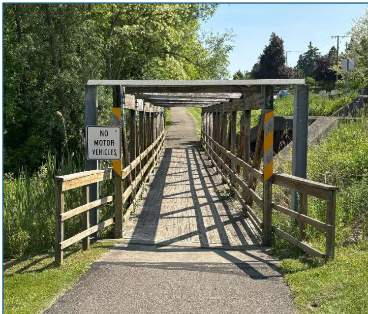
Figure 6.8: Wooden Pedestrian Bridge on Adams Road north of River Trail Drive
