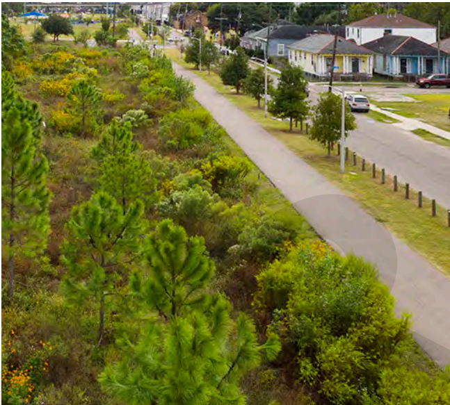
Lafitte-Greenway Bioswales in a flood-prone neighborhood. Source: Brandon Huttenlocher, Design Workshop, Inc.
