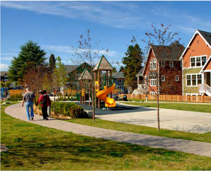
New housing is intended to offer a variety of styles and materials Source: Mithun; High Point Parks - Seattle, WA
