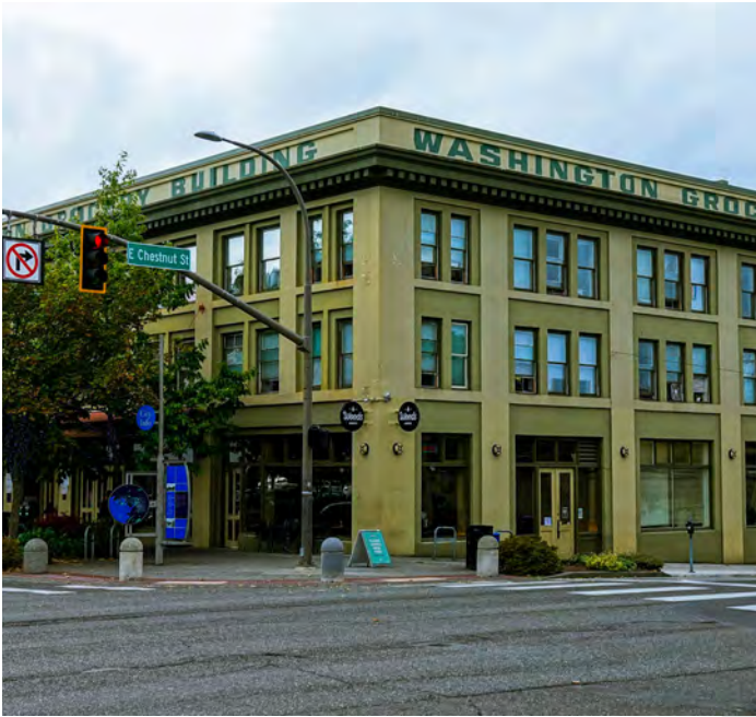
Urban mixed use building with ground floor storefronts.
