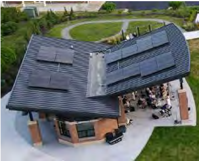
Solar panels installed at Century School Park Source: Verona, WI Website Sustainable Verona Page
