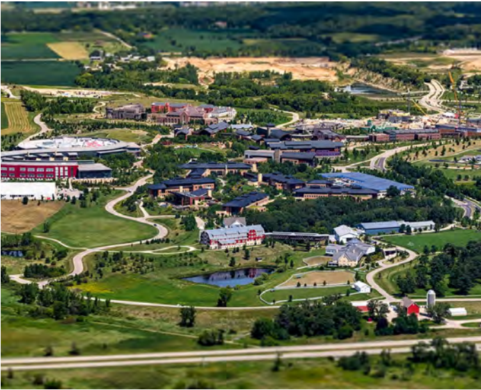
Epic Systems Corporate Campus Source: Epic Systems Corporation
