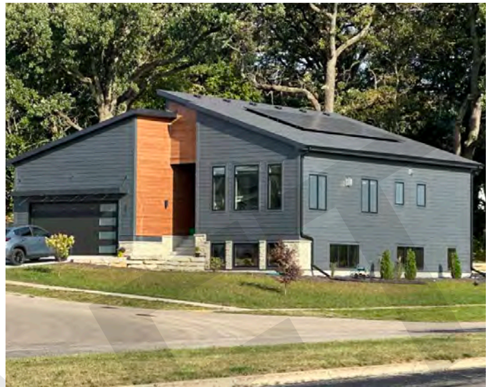
Solar panels on a new private development Source: Sustain Verona
