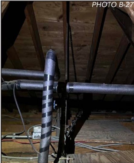
Ventilation Pipe in Attic
