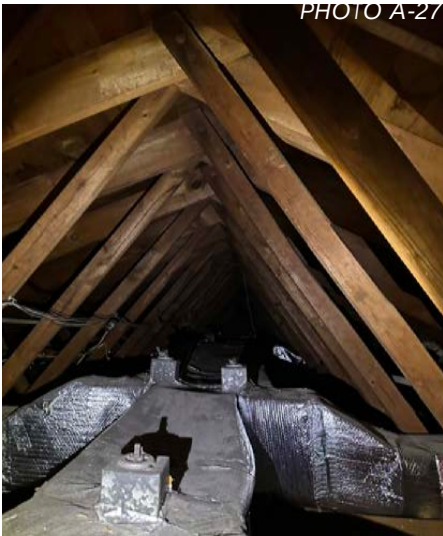
View into Attic
