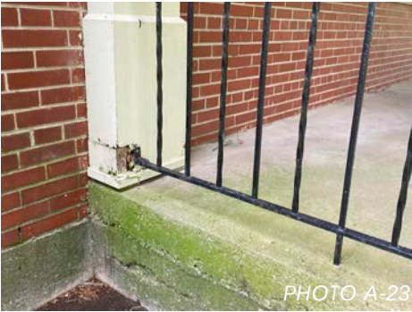
PHOTO A-23 West Porch Column and railing
