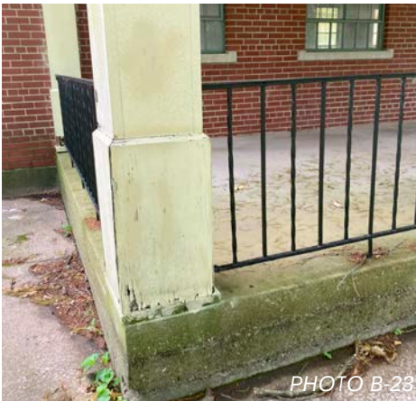
PHOTO B-23 Photo of current wood columns and railings.
