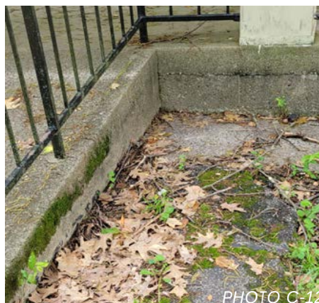
PHOTO C-12 Front Steps, center
