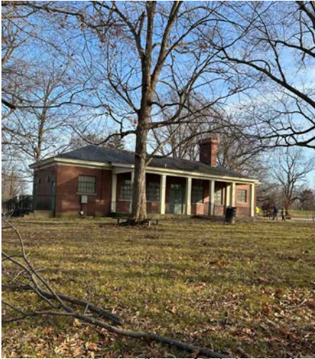
Rear View of Existing Lodge
