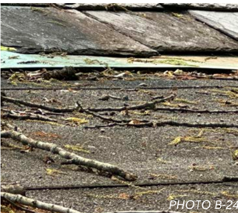
Detail photo of built up roof at South porch
