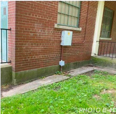
Concrete Apron around Structure
