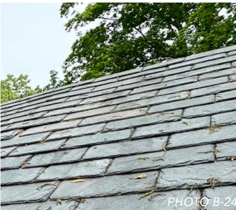
Detail photo of current Slate Roof
