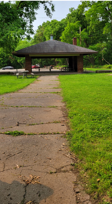
PHOTO A-14 Storm outfall to Ohio River
