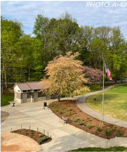
Similar Park Shelter at Tyler Park
