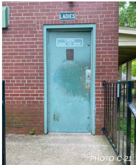
Photo of Women's Restroom Door, Steps and Railing.
