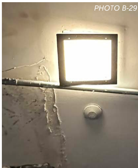
Typical Fire Alarm
