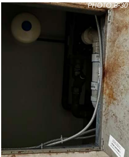
View into Plumbing Hatch In Men's Room
