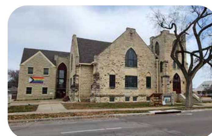
8. First Congregational Church (700 Poyntz Ave; Listed 2008; Significance - Event, Architecture/Engineering; NRR #: 08001068)
