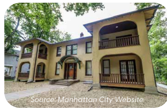
2. The Avalon (417 Fremont; Listed 2019; Significance - Architecture/Engineering; NRR#: 100004453)
