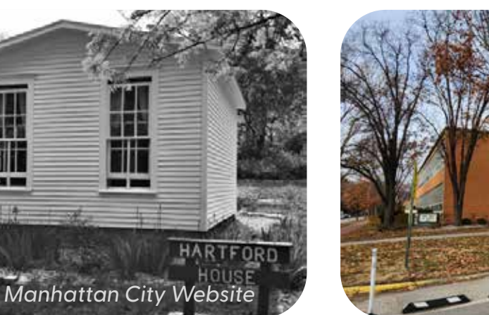
12. Hartford House (2309 Claflin Rd; Listed 2019; Significance - Social History, Architecture; NRR #: 100004452)
