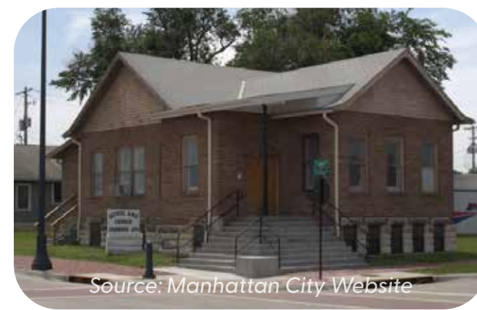
3. Bethel A.M.E Church (401 Yuma St; Listed 2012; Significance - African American Resources; NRR#: 12000301)
