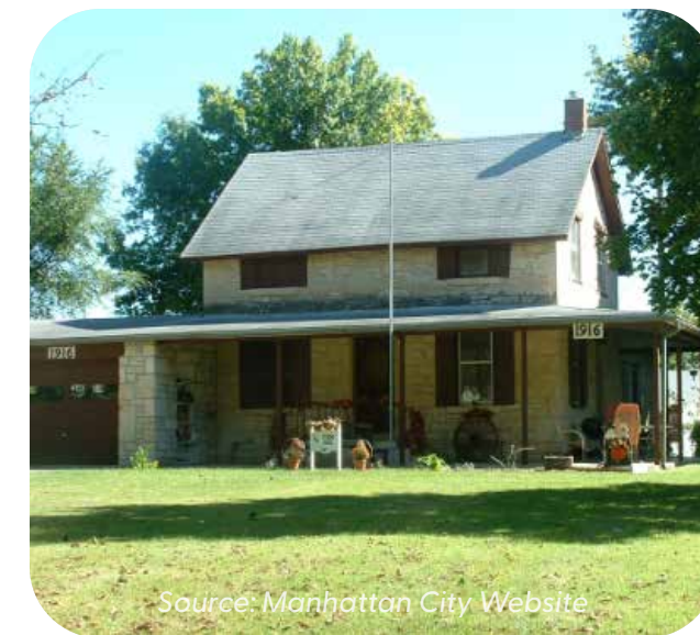
4. Henry and Elenora Strong House (1916 Beck Street; Listed 2009; Significance - Residential; KHRI#: 161-2080)
