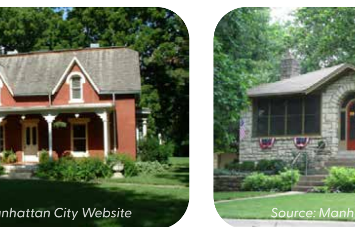
31. Robert Ulrich House (121 North 8th St; Listed 1978; Significance - Architecture/Engineering, Person; NRR#: 78001287)
