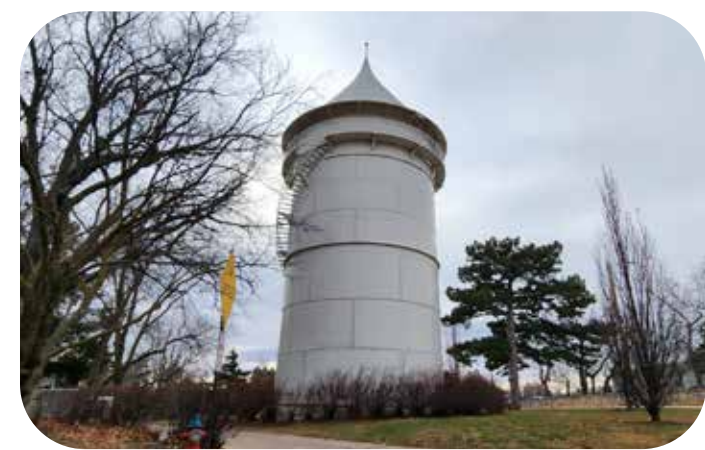
19. Landmark Water Tower (Sunset Ave and Leavenworth St; Significance - Event, Architecture, Engineering; NRR#: 100001704)
