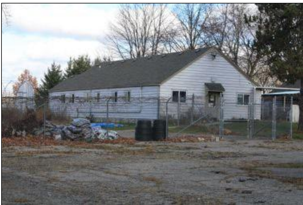
Figure 14. Meadow Brook Poultry Farm, coop 1, view to the northeast
