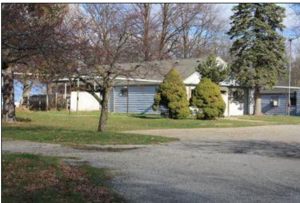
Figure 15. Meadow Brook Poultry Farm, coop 2, view to the northeast
