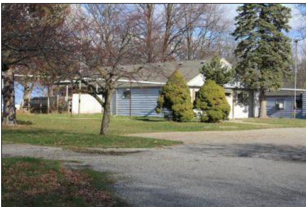
Figure 8. Meadow Brook Poultry Farm, coop 2, view to the northeast
