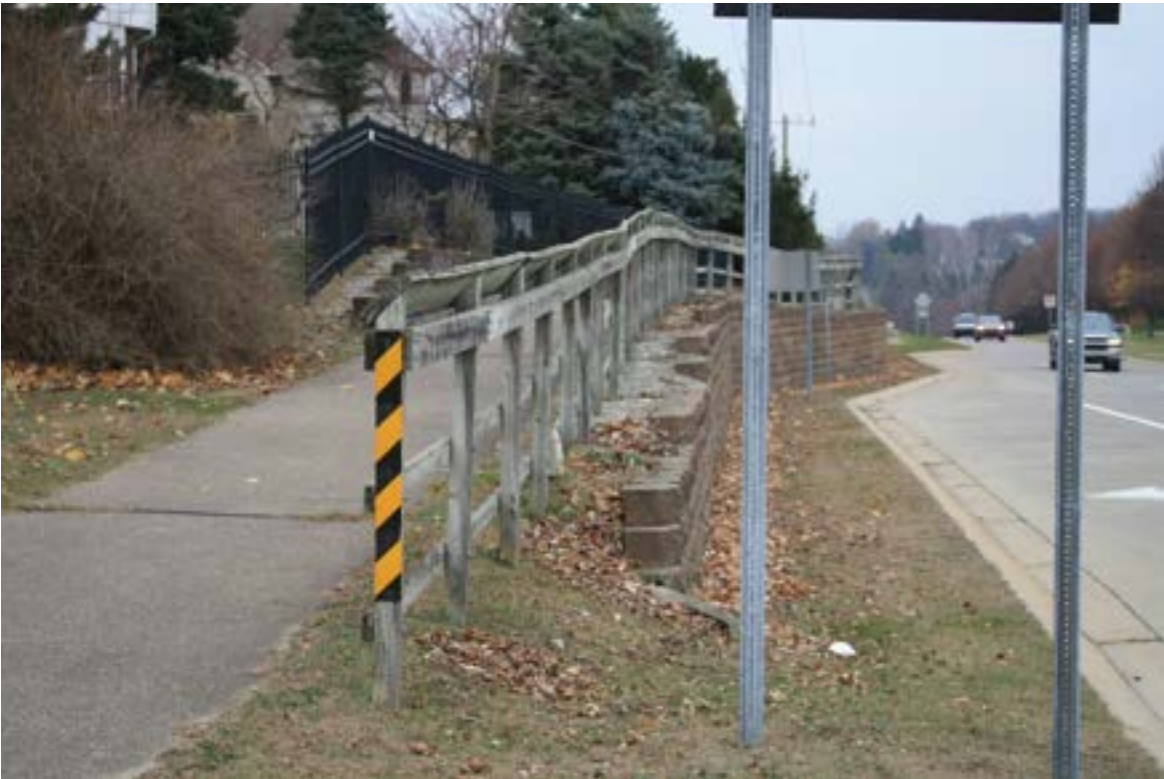
Photo 50. S. Adams Road near the end of the Project Area with non-motorized pathway, looking north.
