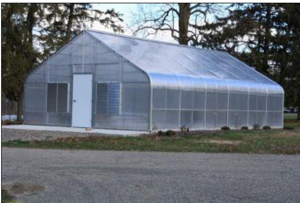
Figure 5. Meadow Brook Poultry Farm, greenhouse, view to the northeast
