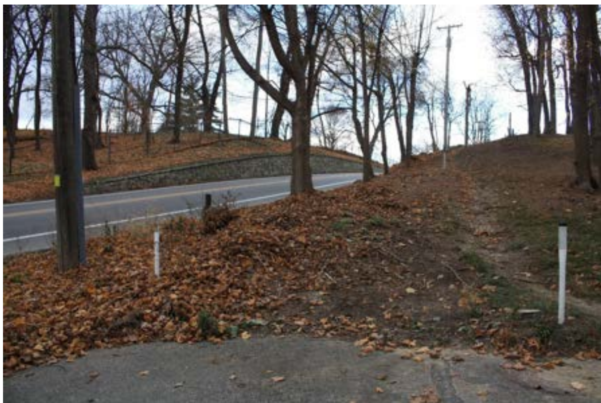
Photo 20. Retaining wall along west side of S. Adams Road, looking northwest.
