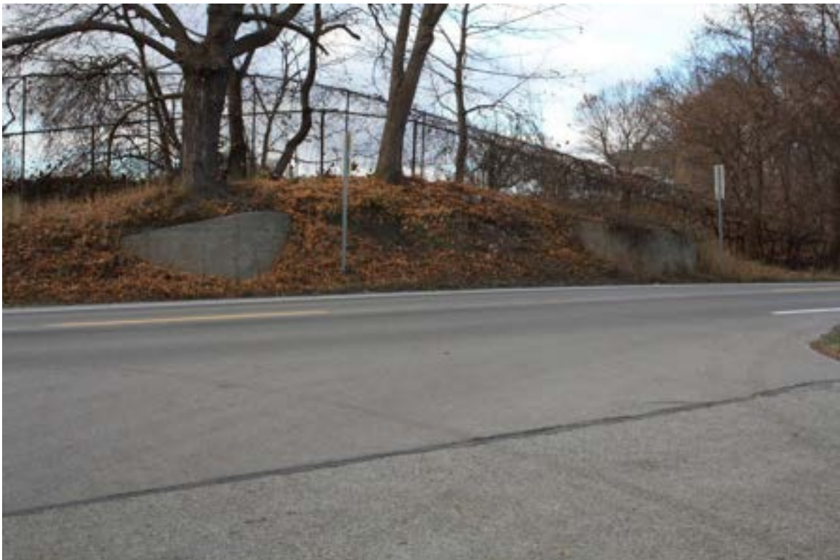
Photo 22. S. Adams Road, Heidelberg Court, and Cambridge Drive, looking northwest.
