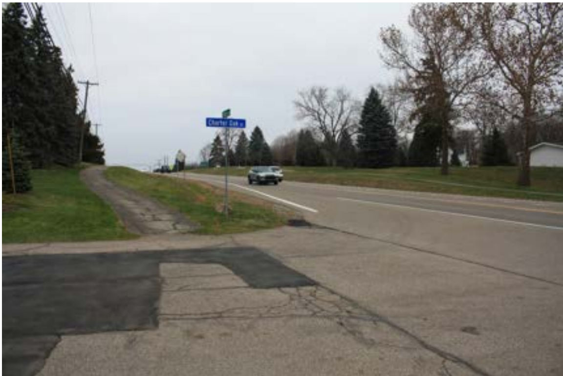
Photo 38. S. Adams Road and Charter Oak Drive, looking northeast.
