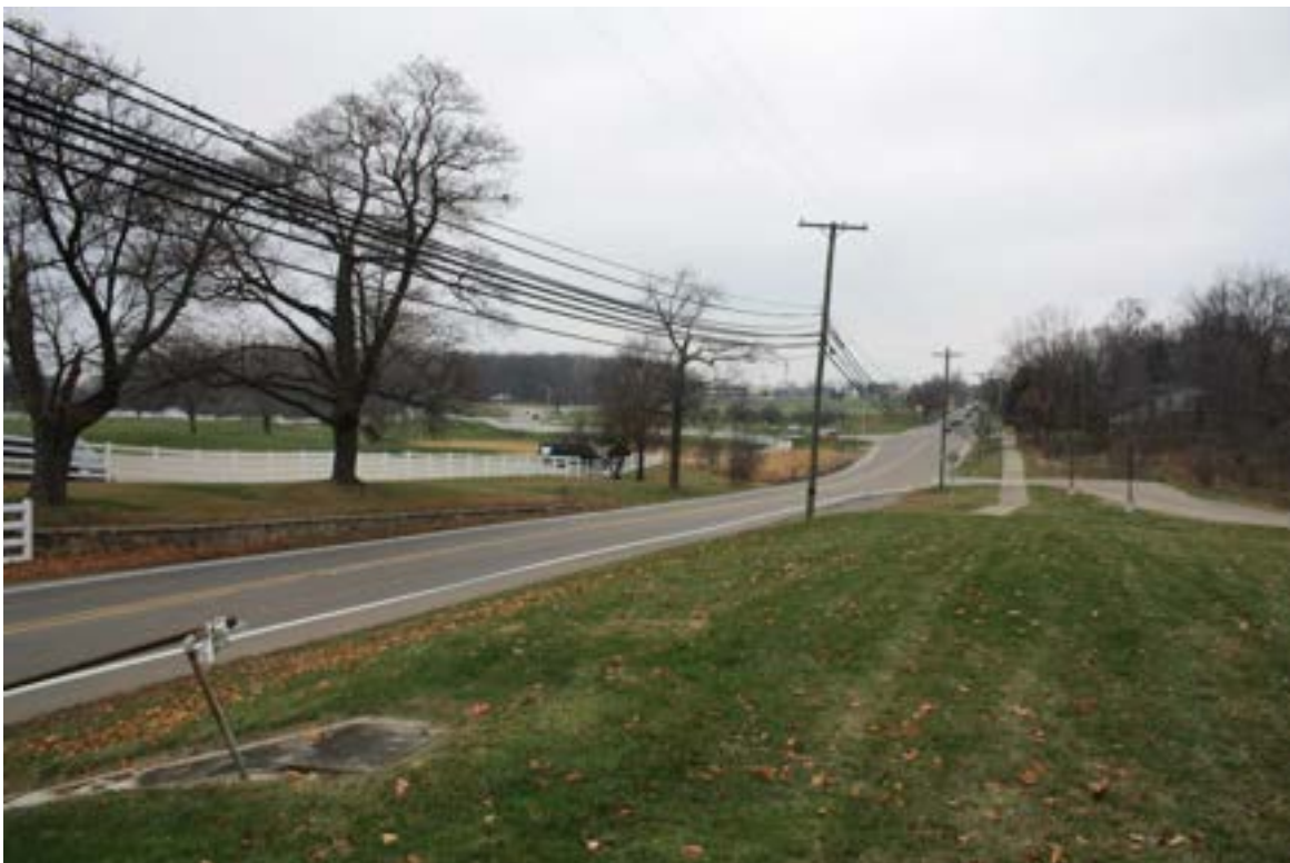
Photo 18. S. Adams Road fronting former worker cottages, looking northwest.
