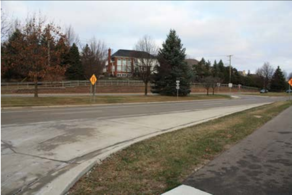
Photo 51. S. Adams Road at southern end of the project area, looking northwest.
