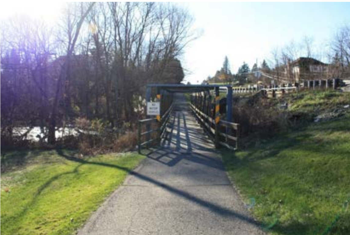
Photo 44. Pedestrian and vehicular bridges over Clinton River, looking south.
