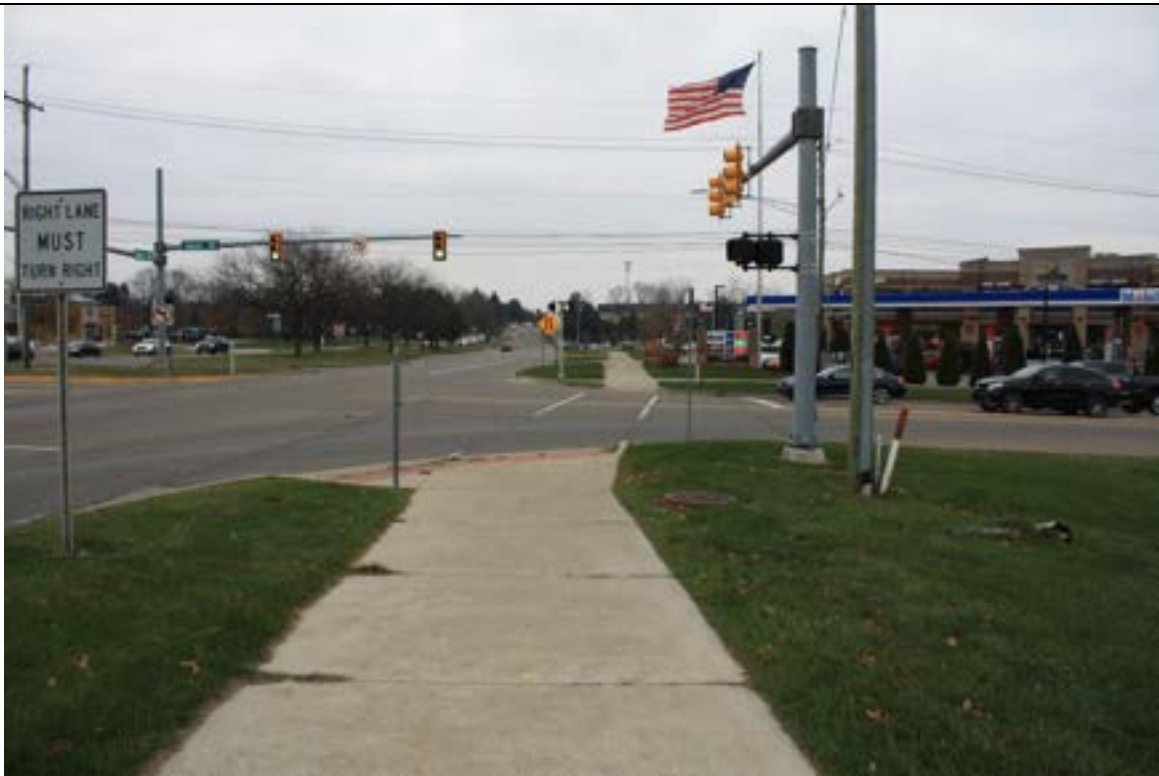
Photo 3. Adams Road and Walton Boulevard intersection, looking northeast.
