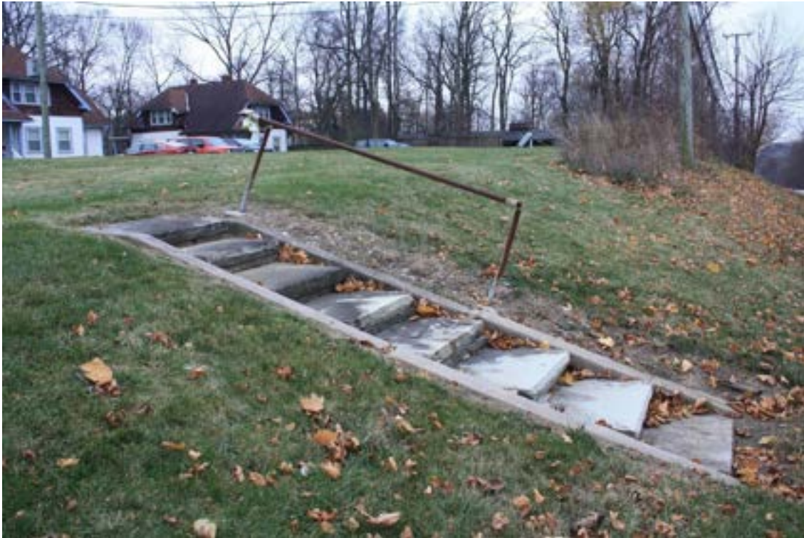
Figure 2-4. Steps leading from worker cottages (in background) to service entrance of Meadow Brook Farms.
