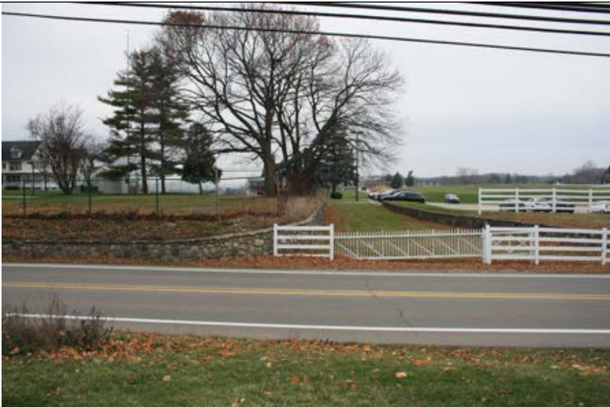
Photo 19. Retaining wall at former entrance to Meadow Brook Farms, looking west.
