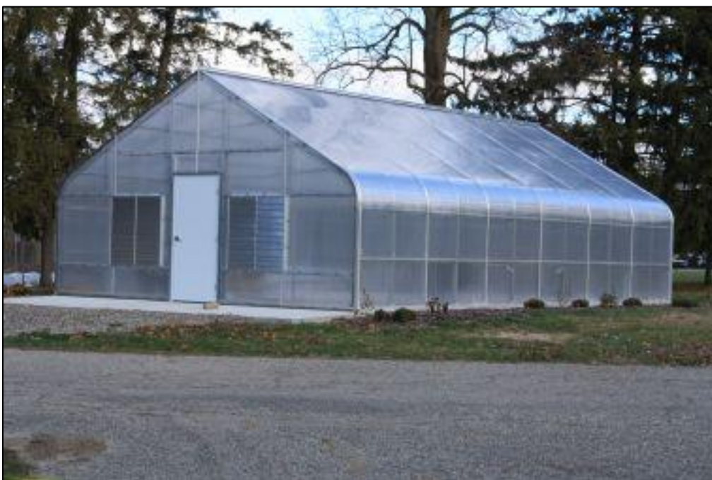
Figure 12. Meadow Brook Poultry Farm, greenhouse, view to the northeast
