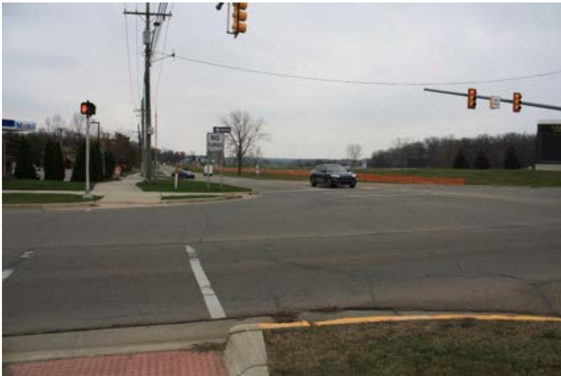
Photo 2. S. Adams Road and Walton Boulevard intersection, looking southwest.
