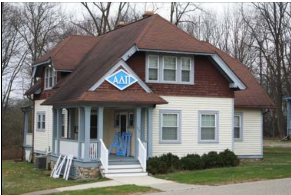
Figure 2. Cottage B at 437 S. Adams Road, view to the southeast
