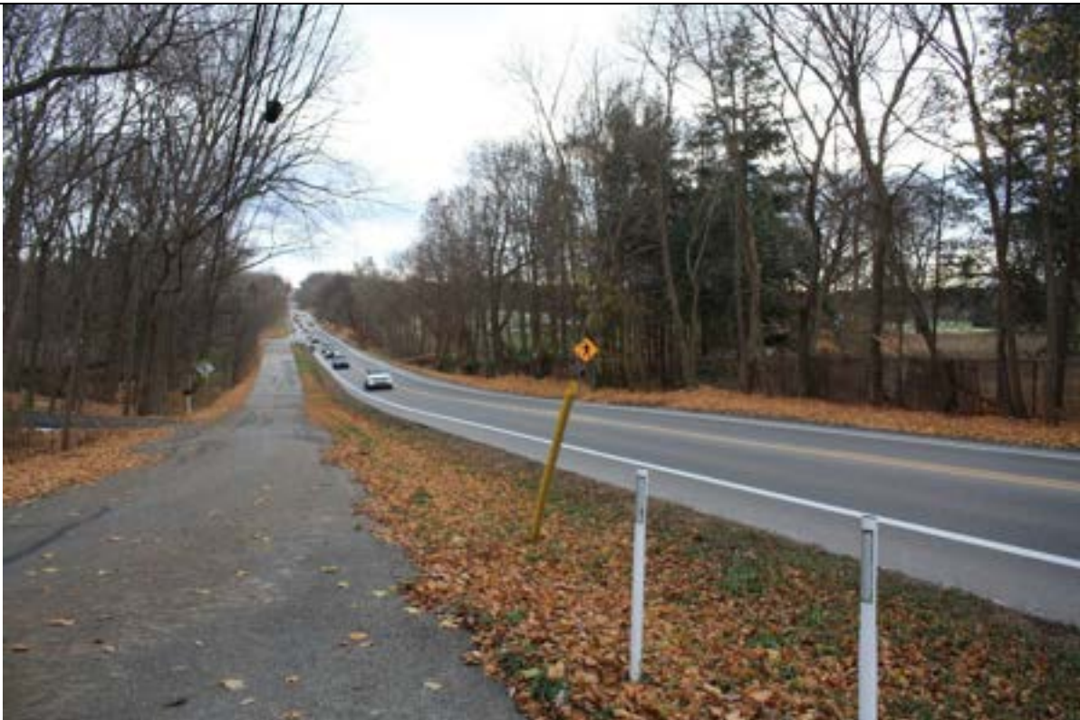
Photo 21. S. Adams Road and Heidelberg Court, looking southwest.
