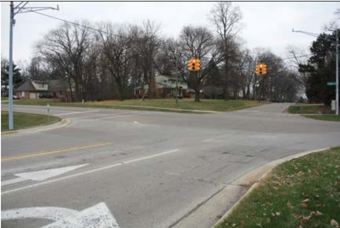
Photo 13. S. Adams Road, Meadow Brook Road and Hillendale Drive, looking northeast.
