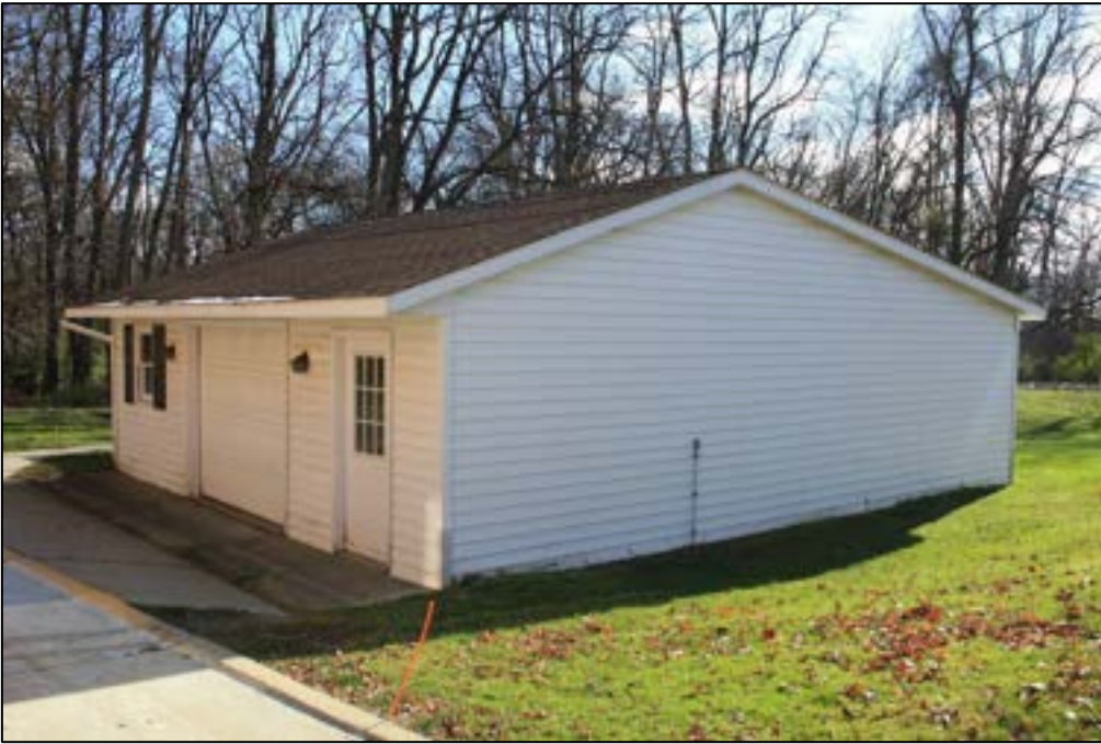
Figure 7. Garage, 1385 S. Adams Road, view to the southeast
