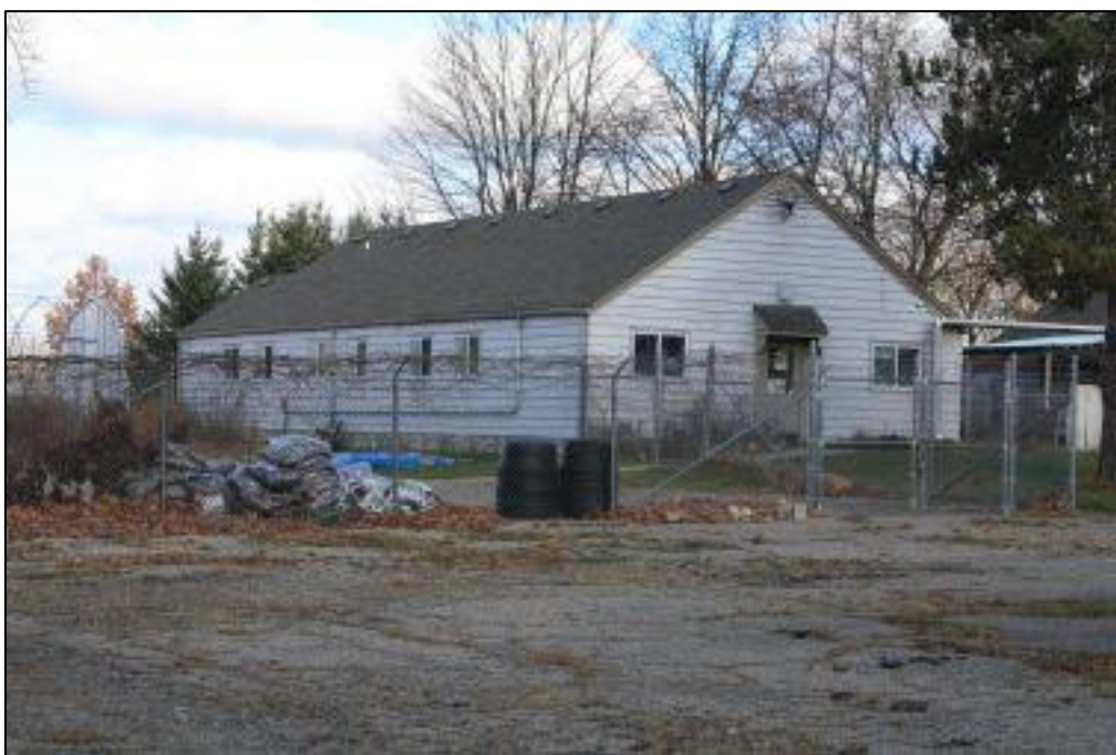
Figure 7. Meadow Brook Poultry Farm, coop 1, view to the northeast
