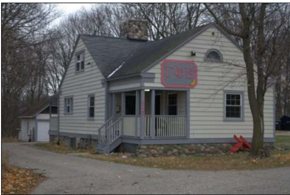
Figure 1. Cottage A and garage at 415 S. Adams Road, view to the southeast
